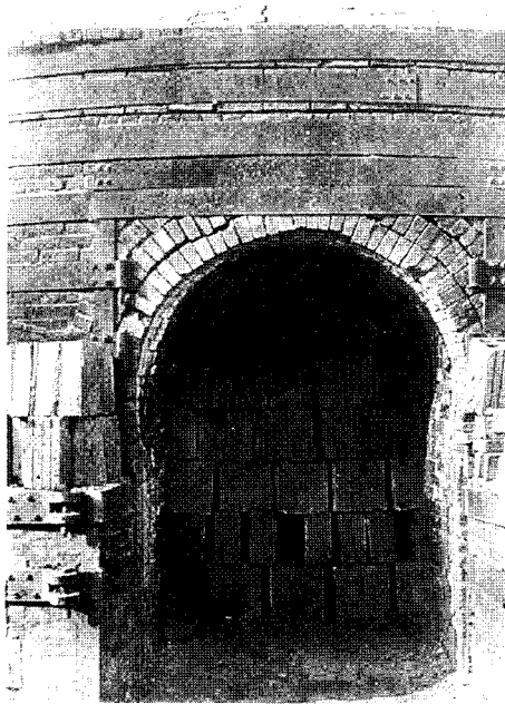
Fig.11. Kiln with previously fired hollow tile blocks (from Squires, The Hollow-Tile House , 5).
